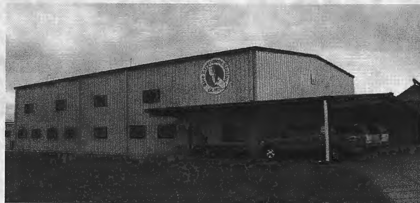
New Research Building
